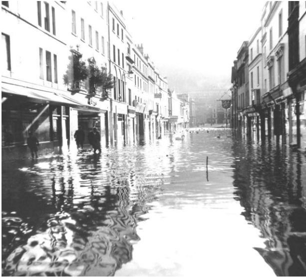
Fig.3 Southgate Street Flooded
